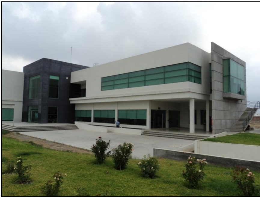
MASTER'S DEGREE BUILDING STAGE II CONSTRUCTION GENERAL CONTRACTOR
