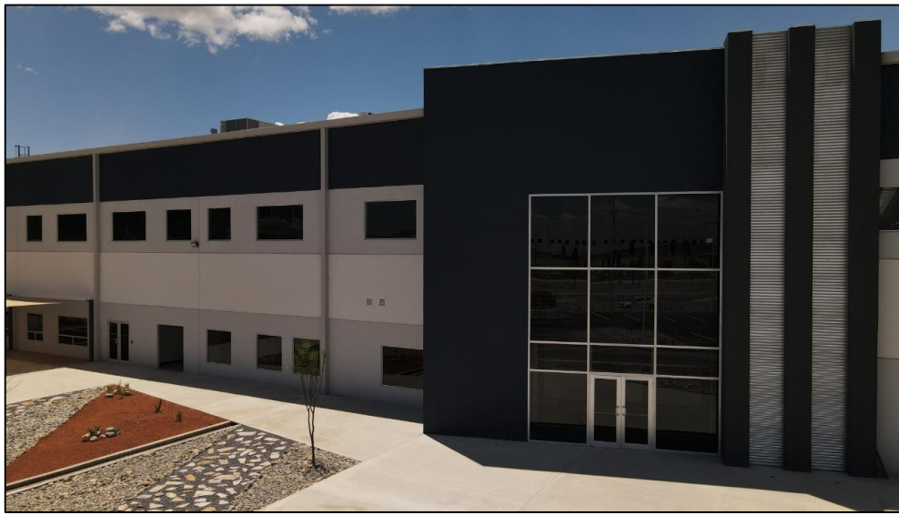
MANUFACTURING BUILDING CONSTRUCTION GENERAL CONTRACTOR 18,000.00 M2 JULIAN ELECTRIC MÉXICO DERRAMADERO, COAHUILA.
