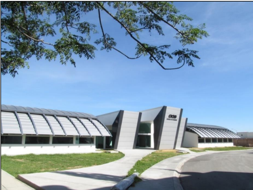
LABORATORY BUILDING CONSTRUCTION GENERAL CONTRACTOR
